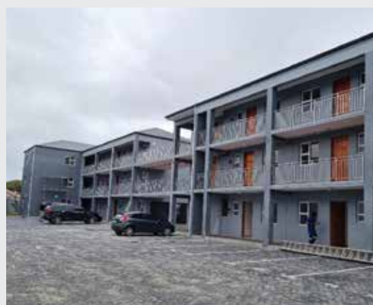
Cape Town Povicom Regent Project
